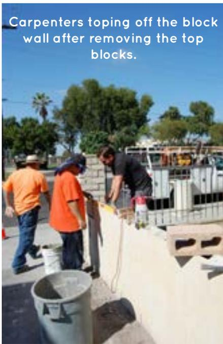
Carpenters topping off the block wall after removing the top blocks.
